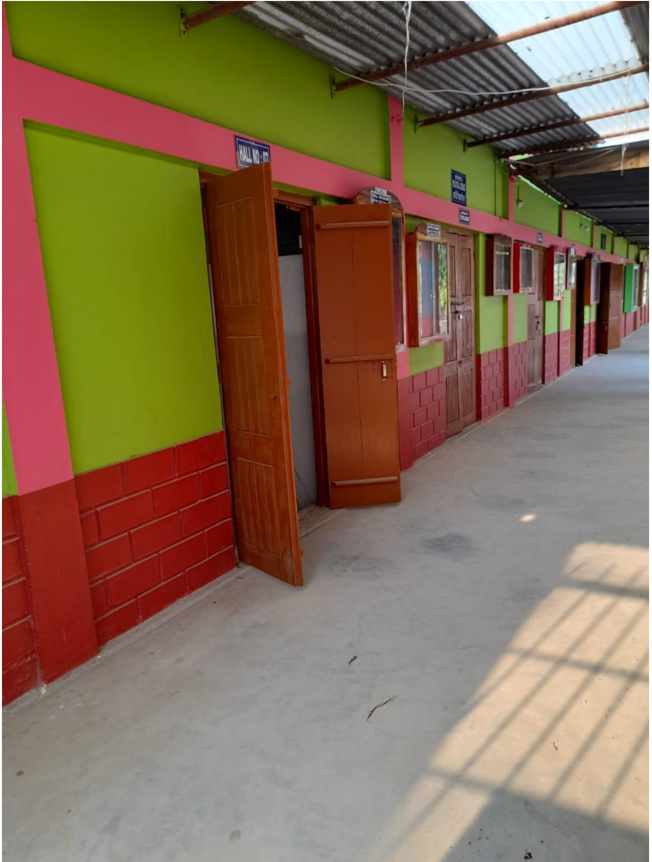
Block-C All Departmental office room & Girl's Common room.
